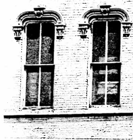
The distinctive features of the Cole Building include cast-iron storefront columns (below) and decorative, terra-cotta window hoods (above).
